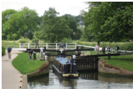
The barge locks at Diglis are listed structures.
