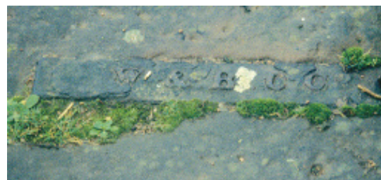
Canal company initials cast into ironwork, Lock 4.
