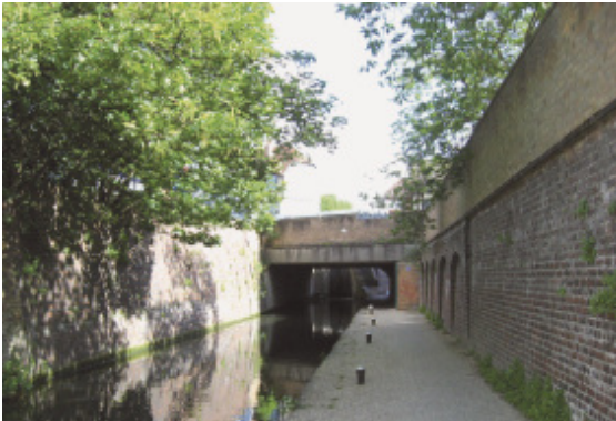
Space is enclosed by the 'cutting' at Sidbury.
