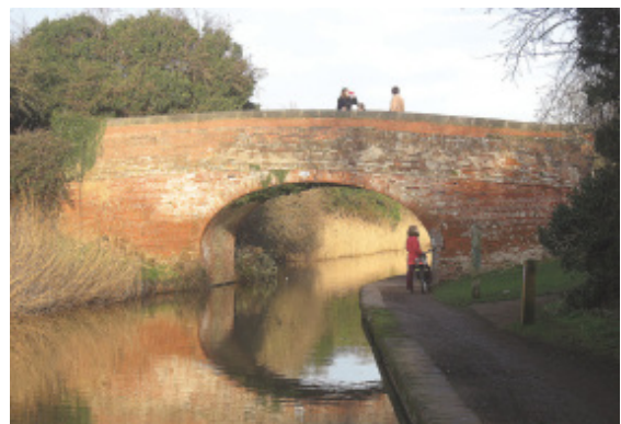
Original brick bridges are locally listed structures.
