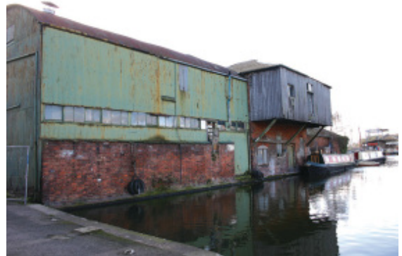
Danks' warehouse in Diglis, in 2006.
