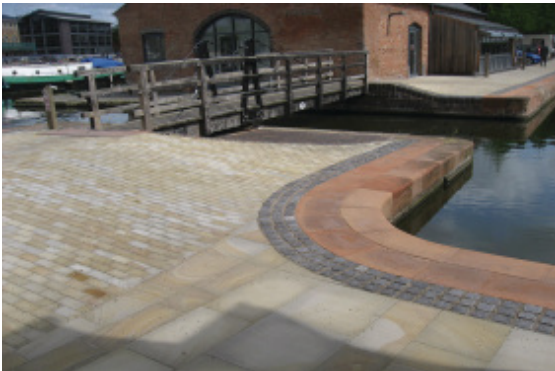
New stone pavings in traditional format enhance the canal-side in Diglis.
