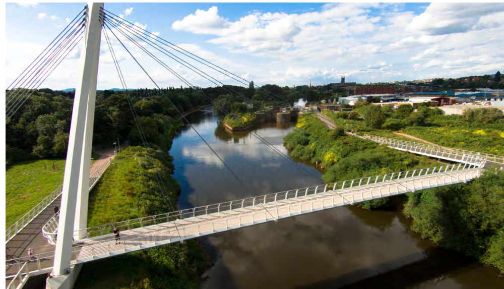
Digilis Bridge. Source: Dronestagr.am Stenweb
