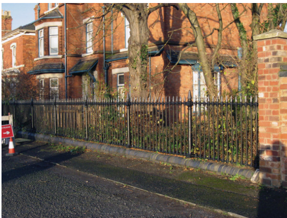
No. 2 Stephenson Terrace.
