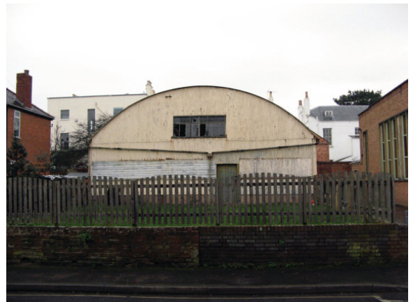
Interesting infill of non-conforming character.
