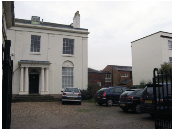
Car parking in front garden - reduces planting, erodes character.
