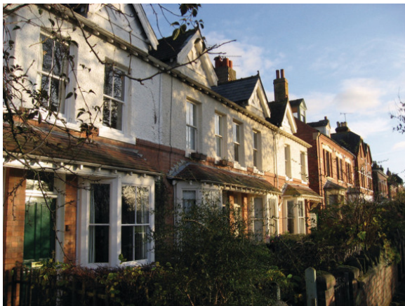
Unaltered details in Stephenson Road.
