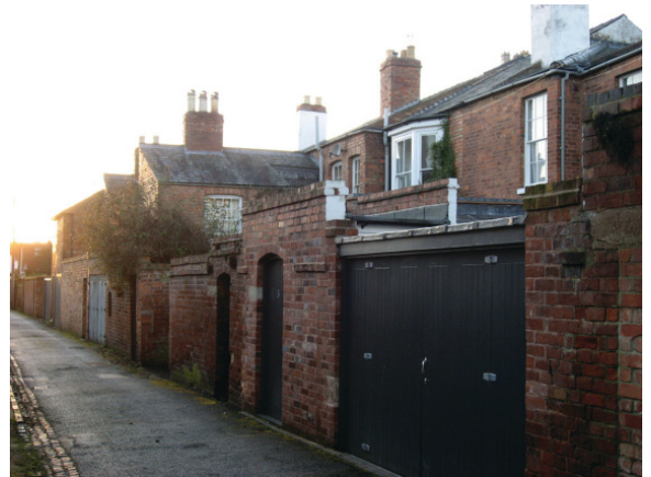
Tight enclosure of space in Back Lane North.
