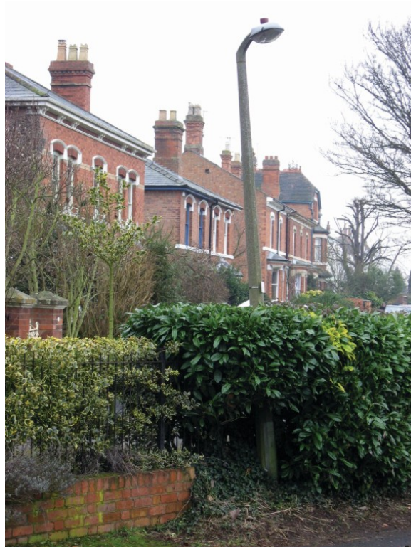
Concrete lamp standard.
