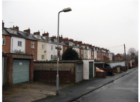
Discordant rear additions to York Place.
