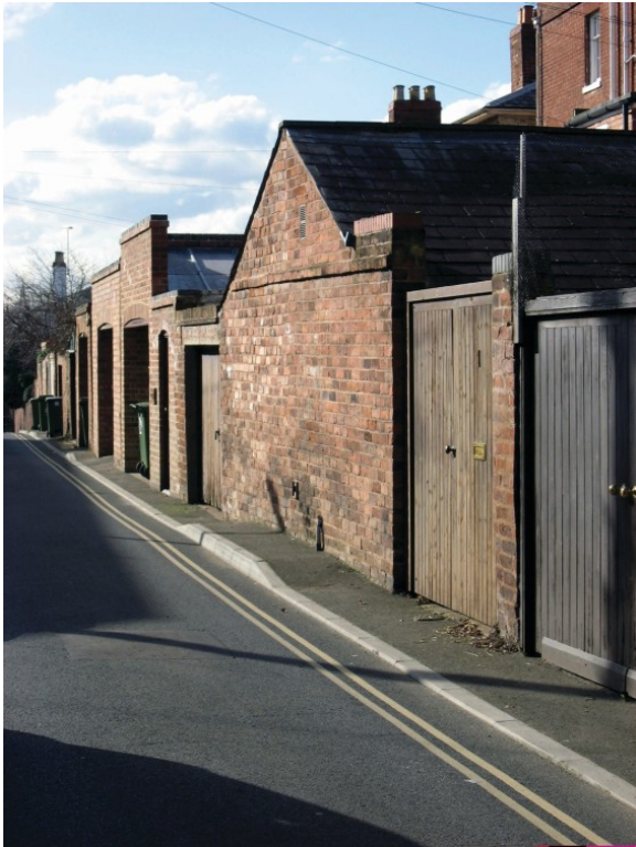
Historic character only on one side of Back Lane South.
