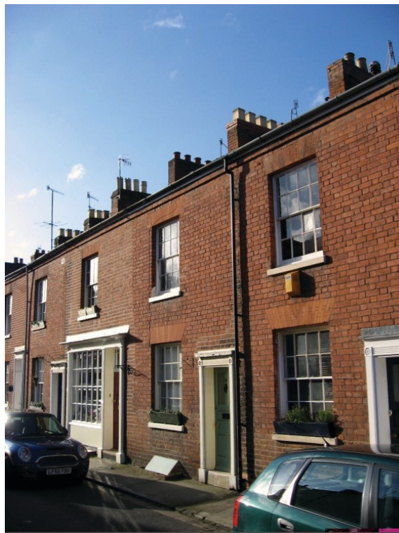
Early shop-front, York Place.
