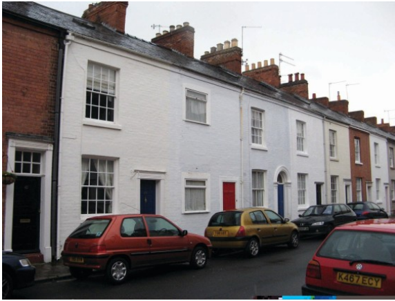
Painted brickwork and altered windows.
