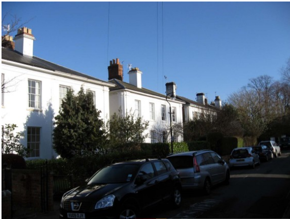
Linked terrace of houses, designed to look separated, on Albany Terrace.
