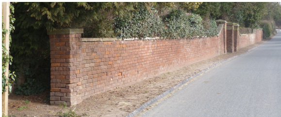
Red brick wall, Church House
