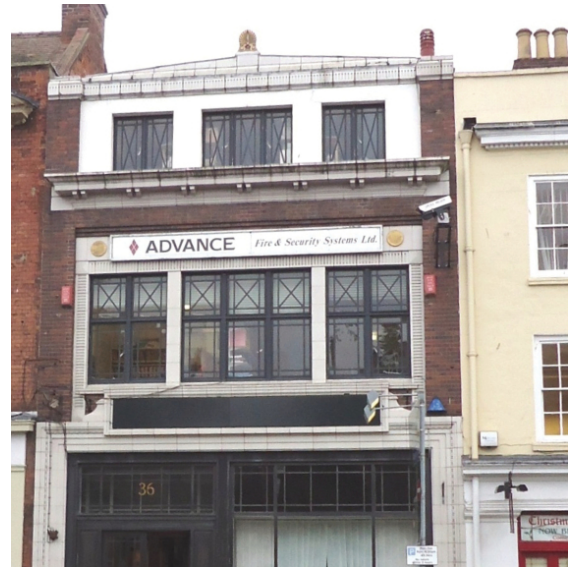
Locally listed, No.36 Foregate Street has white terracotta decoration and metal windows, stylish features of the 1920s.
