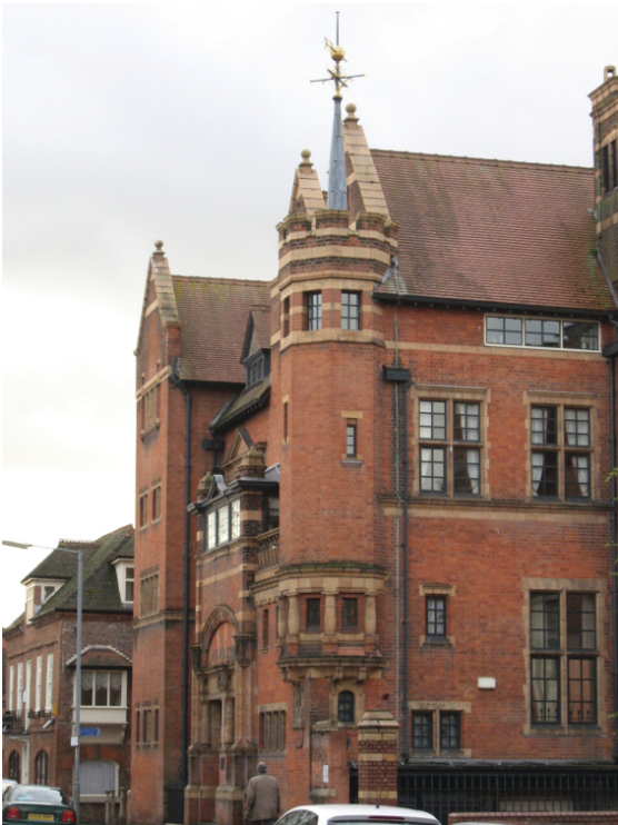
School of Art and Science, Sansome Walk, a grade II listed building.
