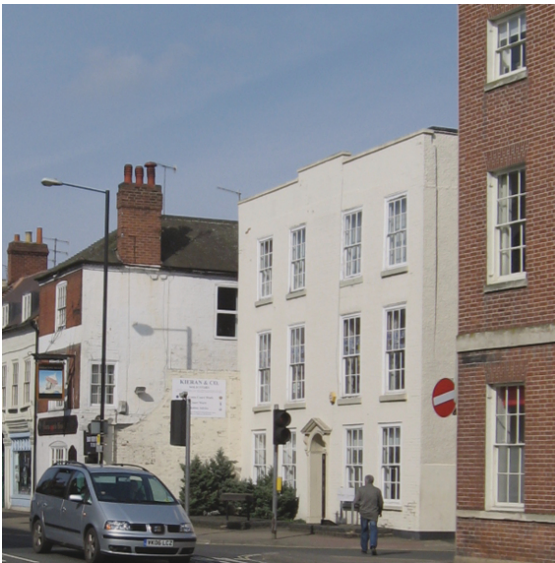
No.1 The Tything is set back from the street, unlike most of the buildings
