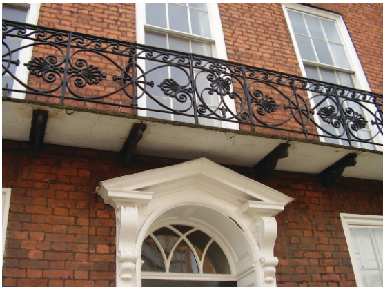
Cast iron balcony front, No.39 Foregate Street
