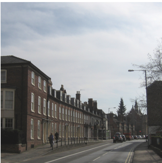
Entering the conservation area from the north, the Georgian character is quickly announced
