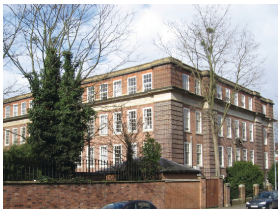
Once an office building for the County Council, this neo-Georgian block is proposed for inclusion in the conservation area.
