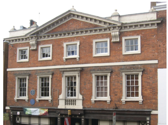
Hastings House in Foregate Street has two blue plaques.
