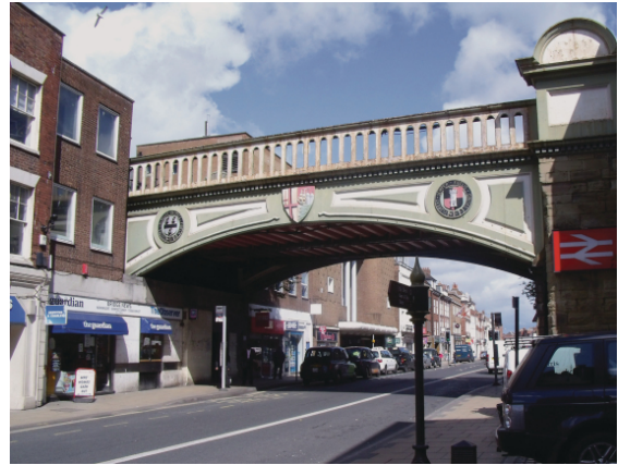
Foregate Street railway bridge is the threshold to the conservation area.
