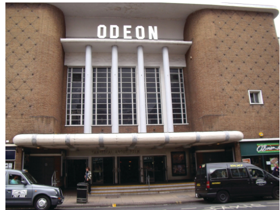
The Odeon Cinema, Foregate Street adds to the diversity of uses.
