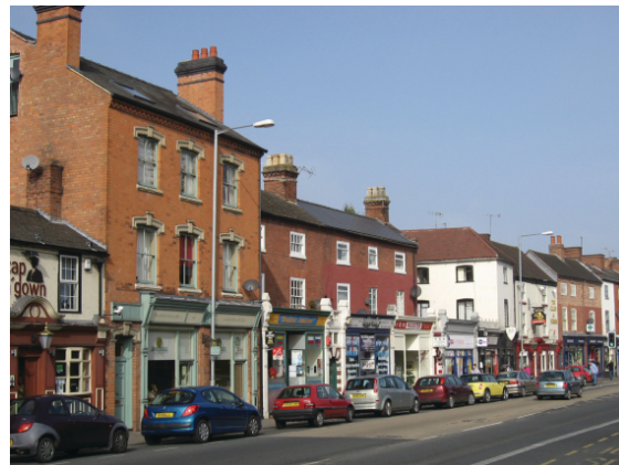
Upper Tything, the west side has a mix of 19 th Century buildings, most of townscape merit.
