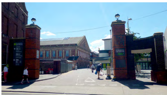
View of Filling Shed from Lowesmoor
