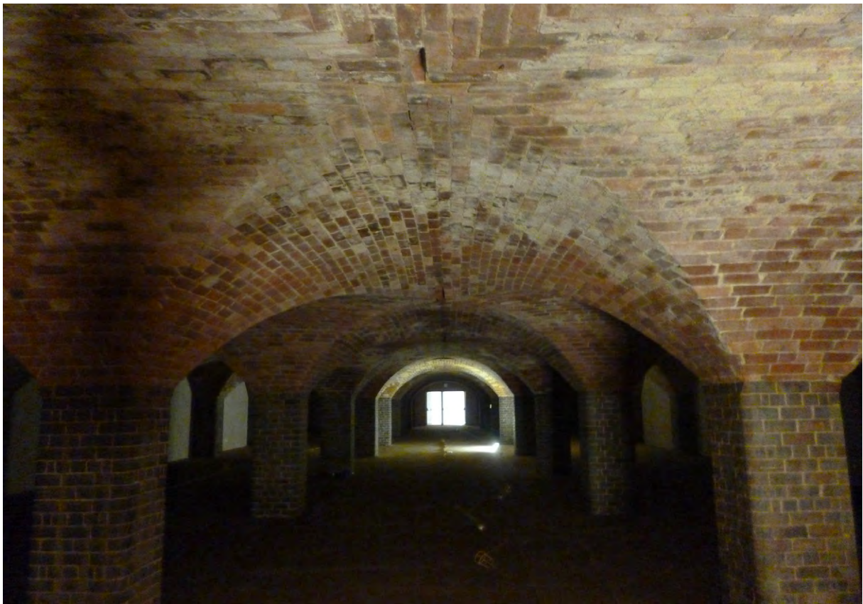
Brick vaulted cellars
