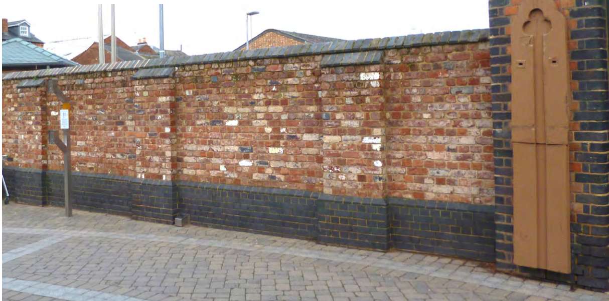
Brick boundary wall, Filling Shed
