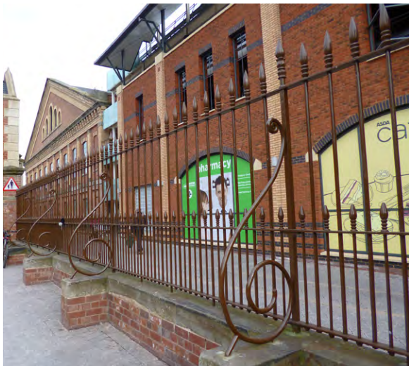
Restored iron railings, St. Martin's Walk
