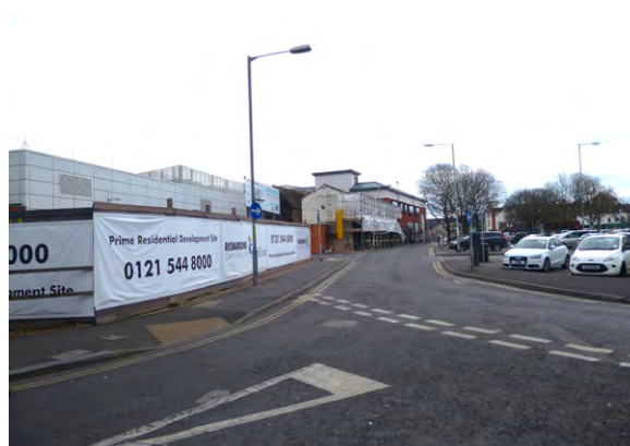
Land clearance to the west of Lowesmoor along Silver Street
