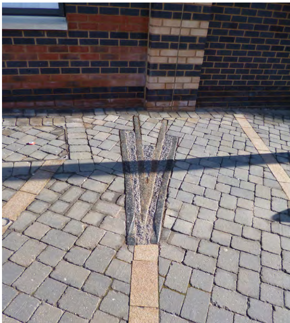
Track lines incorporated into paving scheme
