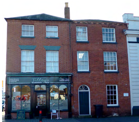
Nos. 64 and 66, Lowesmoor
