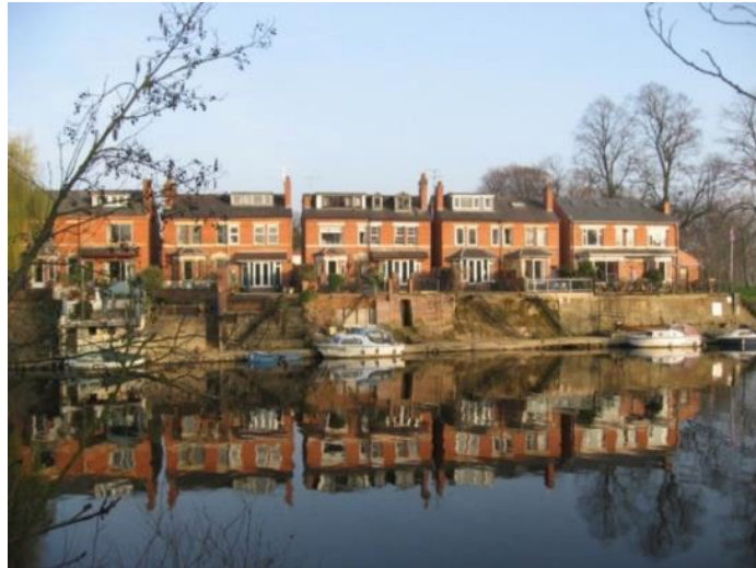
Victorian dwellings on the site of the Pope Iron Works
