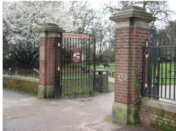
Cripplegate Park Gates
