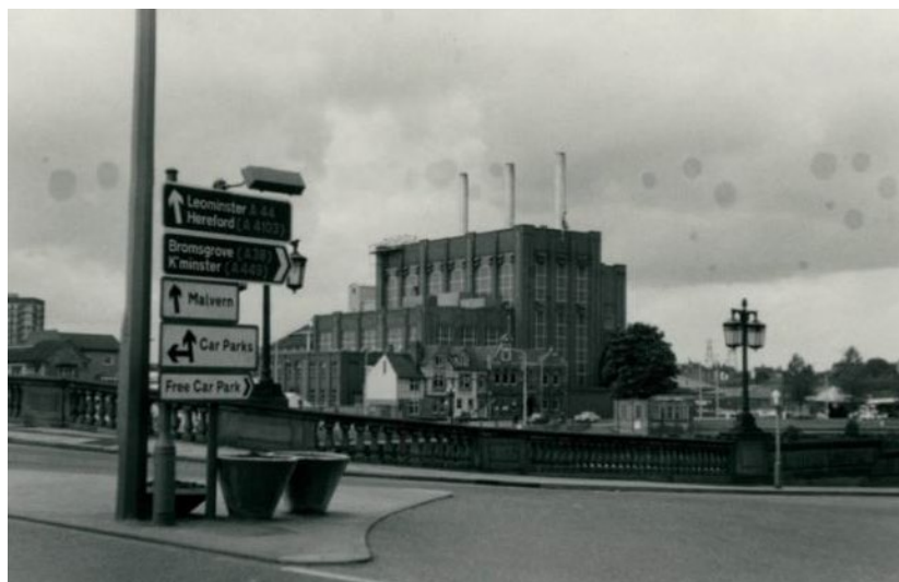
Hylton Road Power Station
