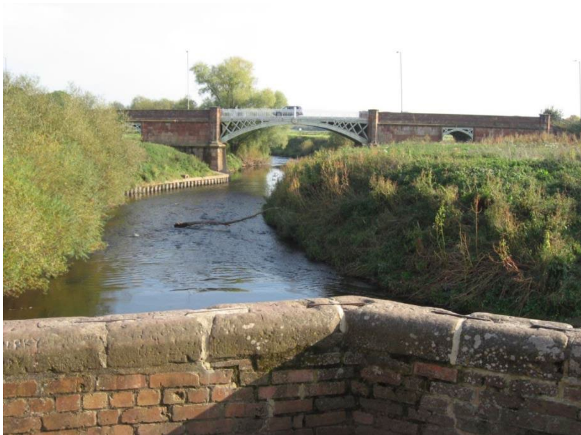
Powick 'New' Bridge from Powick Old Bridge
