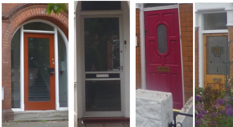
Unacceptable replacement door styles
