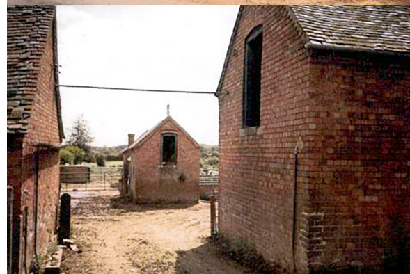
Trotshill farm buildings prior to residential conversion
