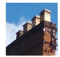
been capped-off or is not used, in order to restore the correct appearance. An open flue provides useful ventilation, essential in helping to control condensation problems. It is recommended that capped flues are provided with through-ventilation to prevent possible dampness in the stack. (NB: Where a stack is capped-off and a pot put on, a gap must be left in the flaunching to prevent rainwater collecting within the pot.
