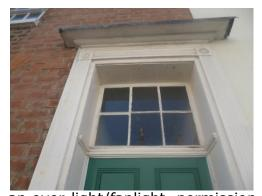
Where there is no fanlight (semi-circular window) or over-light (rectangular window) above the door, the top two panels of the door could be replaced with six millimetre float-glass but this is a non-preferred alternative and does have repercussions on security and privacy. The glass can be clear or obscure either by being ground or lightly textured such as 'Stippolyte'. Where there is
