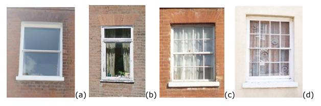
For example a traditional (a) or modern (b) replacement window can be restored to an eight-over-eight timber sash window (c) but a uPVC sash window would not be acceptable. Replacement glazing (d) which alters the character of the window will not be acceptable and sash horns should be avoided.
