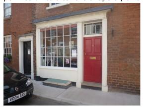
correct recess depth of  $114mm (4\frac{1}{2}")$  from the outer face of the brickwork to the front face of the wooden sash frame must be retained.
