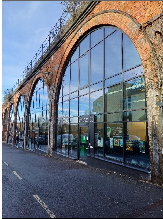
Image 16 Shop frontages within Railway Arches
