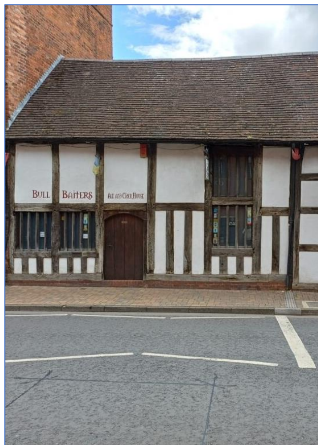
Images 3-4 examples of existing timber framed buildings including shopfronts
